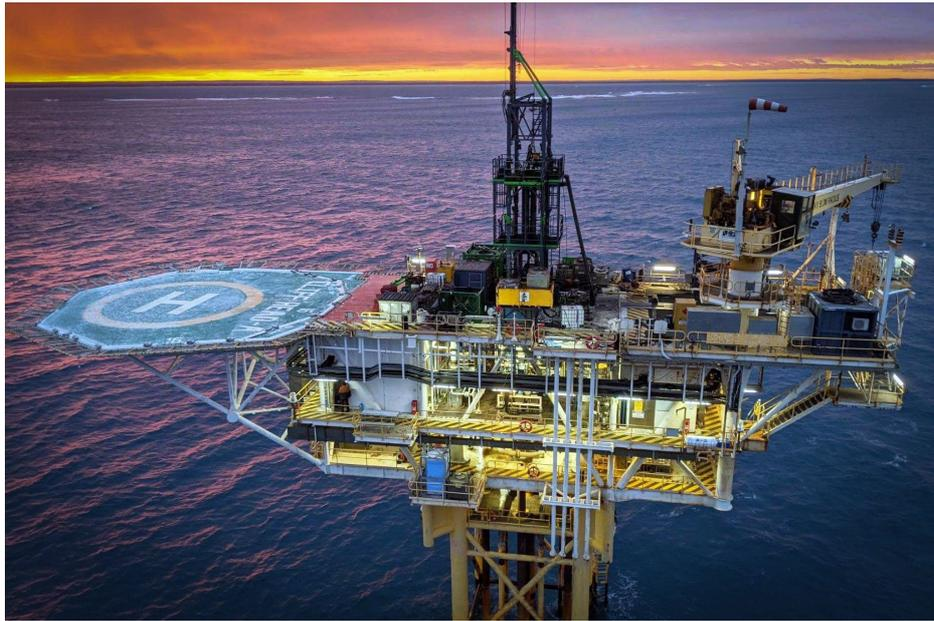
Cliff Head Alpha platform with Hydraulic Workover Unit installed
