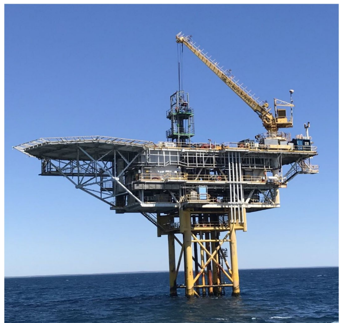
The recently commissioned Hydraulic Jacking Unit at Cliff Head Alpha
