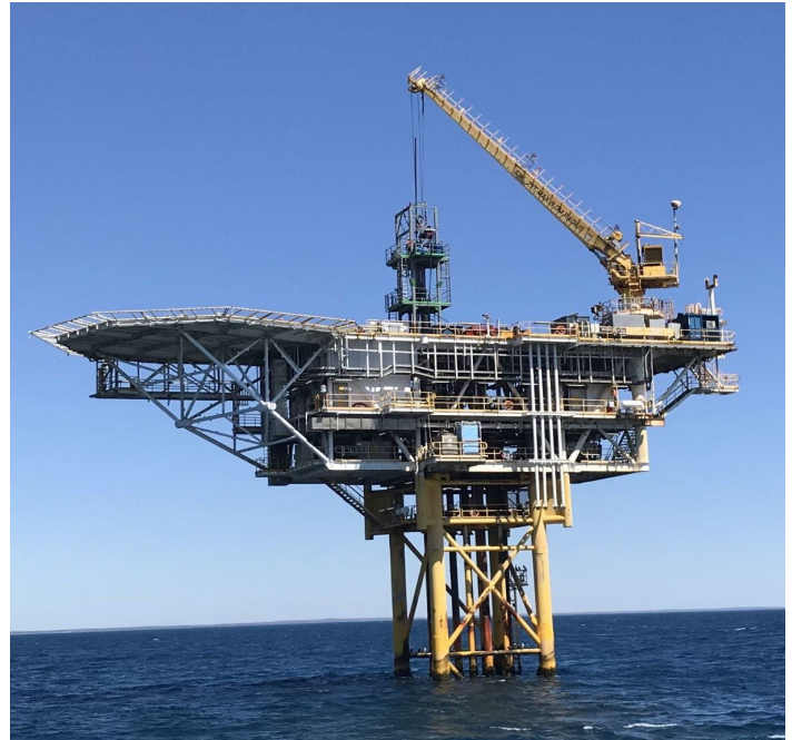
Figure 2: Cliff Head – The Cliff Head Alpha platform with the workover unit installed
