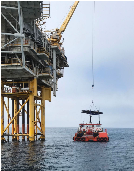
Figure 1: Unloading tubing from the Supply Vessel
