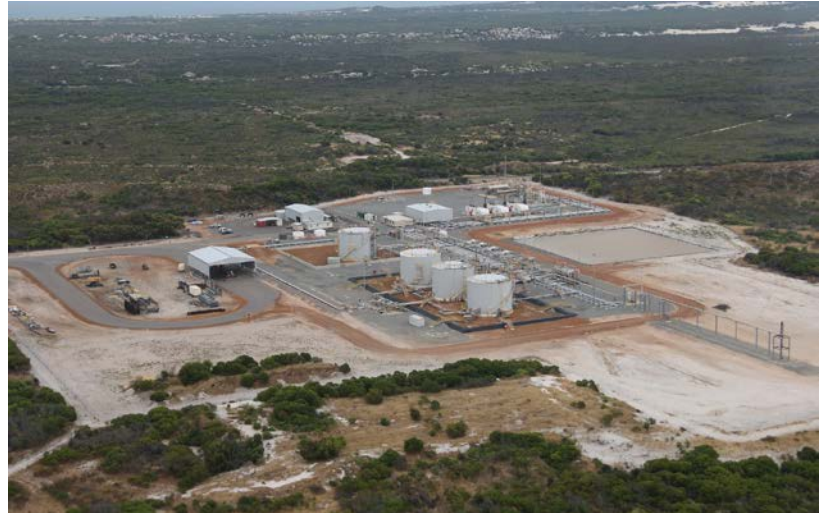
Arrowsmith Stabilisation Plant
