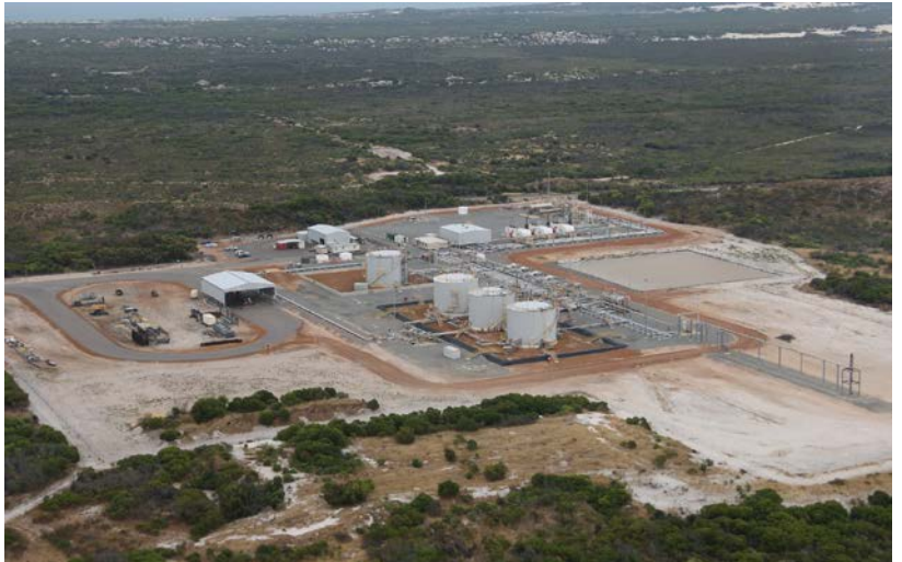
Arrowsmith Stabilisation Plant
