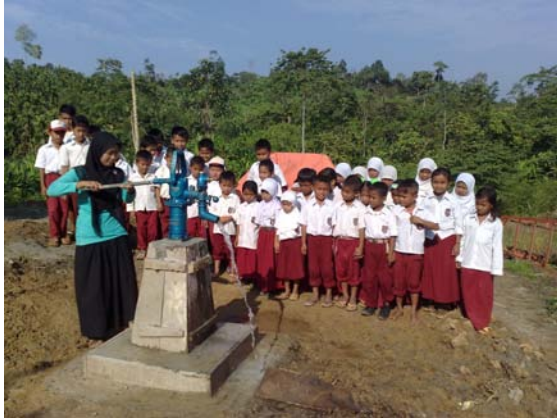
Figure 4 Completed water pump at local school
