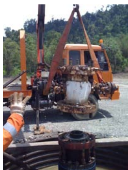
Figure 3 Removal of A-2 well head spool, to prepare for A-2 workover
