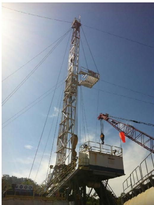
Rig#88 Skytop Brewster has undertaken drilling of temporary cement plugs from Pase A-2 to a depth of 7403 feet. Once total depth is reached Triangle Energy will commence installation of new 4 ½" Chrome completion tubing.
