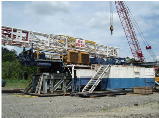
Figure 1 Rig substructure at A2 location
