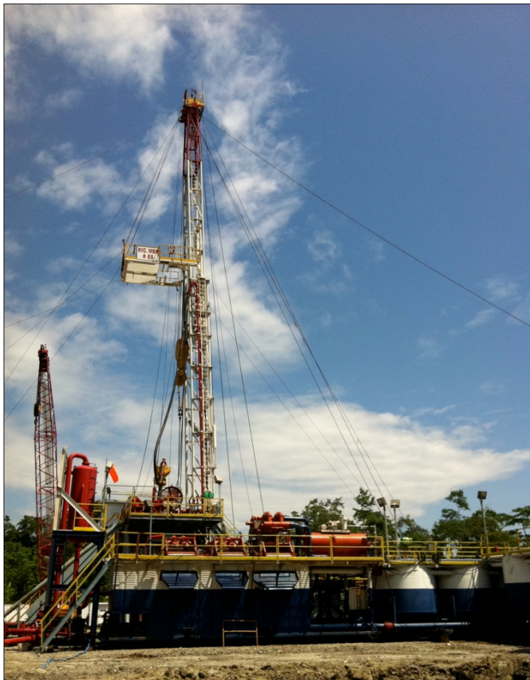
Figure 1 Rig #88 rigged up on location at Pase A-2
