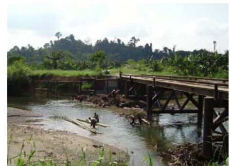
Bridge to A-8
