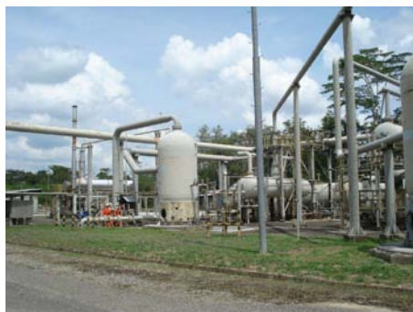
Pase A Production plant
